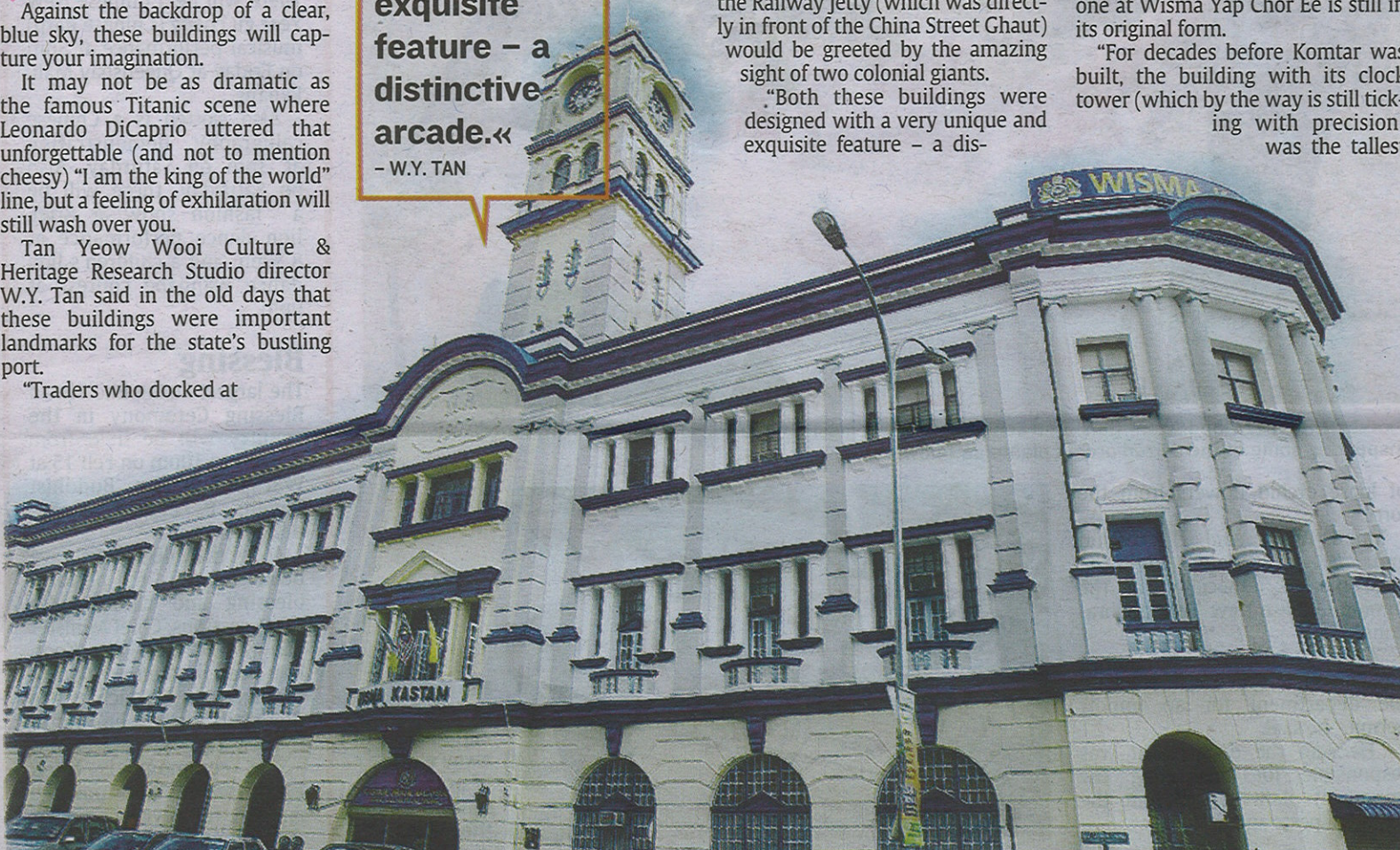
Majestic: The Malayan Railway Building or Wisma Kastam as it is known today.
